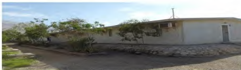
Engineers and clerks dormitory
