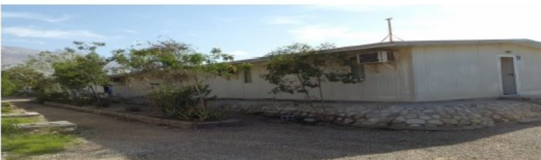
Engineers and clerks dormitory
